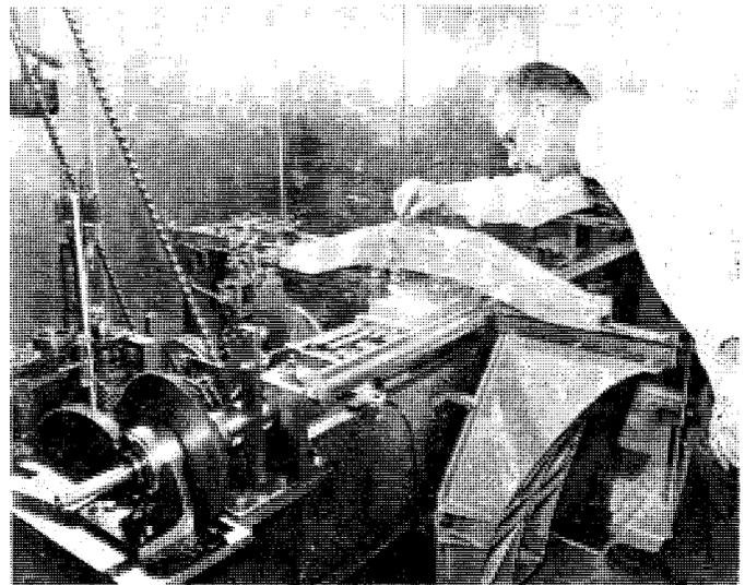
**Fig. 3.** R. S. Wiley is adjusting the diamond during the 8 to 60 setting up hours on the Chicago engine at B & L. To the left of the lead screw, just before the large spur gear is the cylindrical cam on which a follower rests. Prepared interferometrically, this cam corrects for errors in diamond placement to reduce ghost intensity. The gears may be so combined that almost any spacing can be achieved. (Courtesy B&L.)
